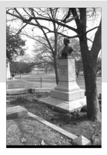
Careful planning and the proper equipment should be used when moving headstones and curbing. Stones can weigh up to 165 pounds per cubic foot. Here, the curbing of the Wharton Monument at the State Cemetery in Austin undergoes restoration.
