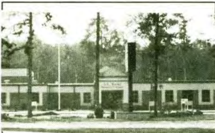
A. R. Turner Elementary School
