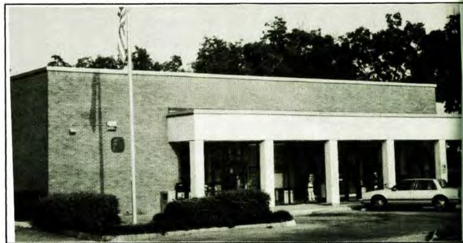
Willis Post Office at Campbell Street location.
