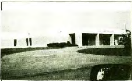
Mel Parmley Elementary School (formerly Willis Elementary School)
